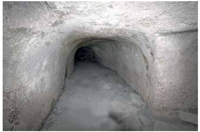
Fig. 9 – The large straight basket vaulted gallery, 21 m long, which connects to the church (photo A. Yamaç).
