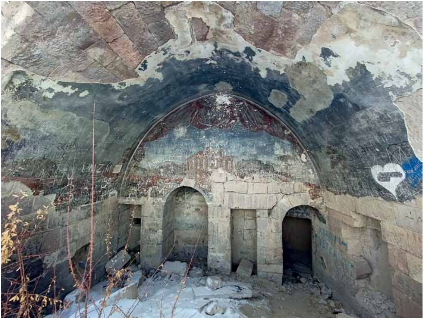
Fig. 11 – Niches and frescoes in the chamber (E), entirely built with ashlars and a pointed (two-centered) vault, claimed to be a chapel (photo H.I. Kala).
