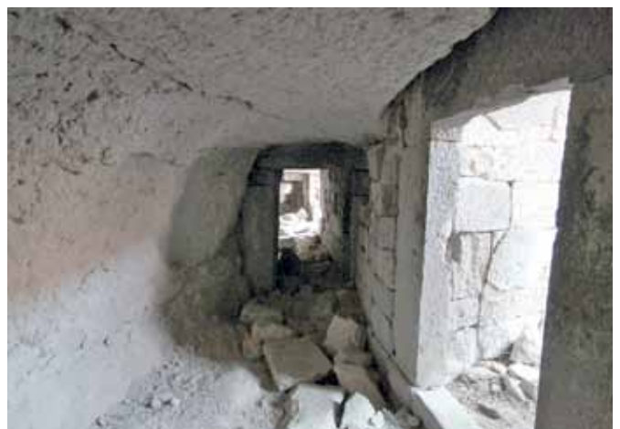
Fig. 10 – The doors of the chambers along the longitudinal flat-ceiling corridor (D). One can note the walls partially composed of squared stones, as well as jambs and lintels made from monolithic blocks (photo A. Yamaç).
